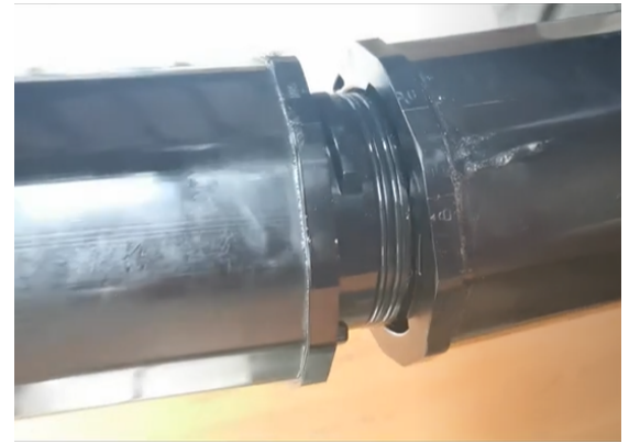
Connect the two shower body pieces and tighten them securely.
