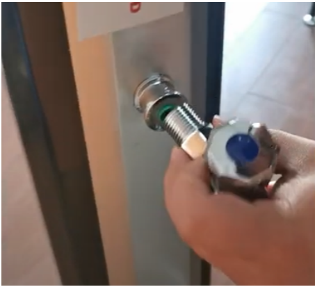
Screw in the faucet piece. Make sure the spigot part where water comes out is facing downward.
