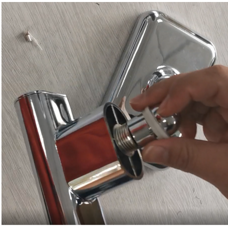
Screw in the connector piece inside the shower head base. Attach the shower head and screw into place.
