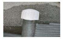
6. Plug return fitting in pool to ensure no water loss when disconnecting hose from return.
