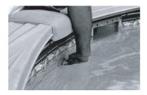
7. Make sure filter is turned off so no water flows out of the filter when disconnecting return hose from the swimming pool return and connecting to the solar heater.
