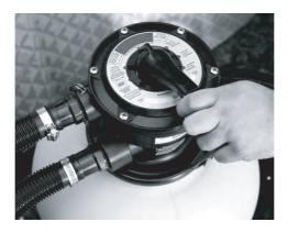
8. Secure flex hose to the top PVC elbow and return fitting of the pool using the stainless steel hose clamps.
