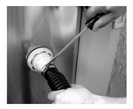
9. Remove the plug from return fitting and turn on the valve for the filtration system, and make sure water flow is freely in all the piping.
