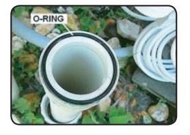
**Step 6.** Inspect the O-rings inside the union connected with the pipe for any wear and replace them if possible. Apply a thin layer of lubricant to the O-ring.
