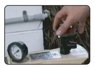
**Step 2.** Relieve the water pressure at the relief valve, it is usually on top of your pool filter.
