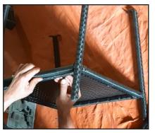
**Step 2:** Lay the table top panel flat on a level surface and line up the assembled portion of the table to the top panel. Affix with bolts and tighten.
